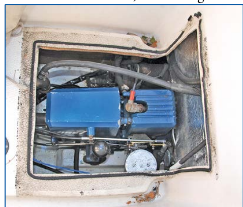
Brygggrannens Vire motorinstallation.
